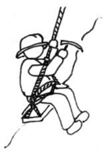
15. Mountains: Railroad tracks could only have a 2% gradient in the mountains. For every one hundred feet, railroad tracks could rise only two feet or the heavy train would slide back down the mountain. Workers had to chip away the sides of the mountains to make a road for the tracks. They were lowered with ropes to drill holes. Then they had to insert explosives and light them.
